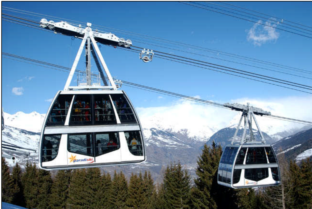
Figure 3.3 – Poma TRASSE in Paradiski France
