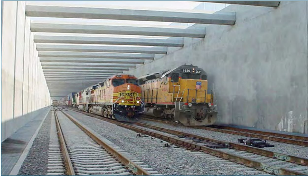
Figure 3.6 The Alameda Corridor
