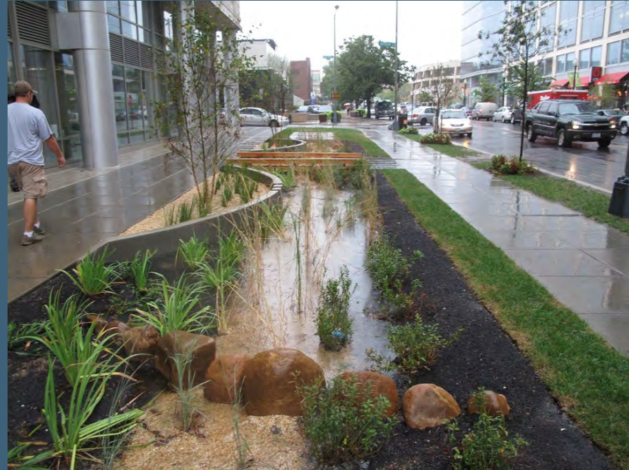
City of Hermosa Beach received CalTrans Sustainable Transportation Planning Grants: Adaptation and Planning Grants to develop a Constraints Analysis and Conceptual Design Project for a suite of green infrastructure and sea level rise resiliency improvements. Photo for illustration purposes only.
